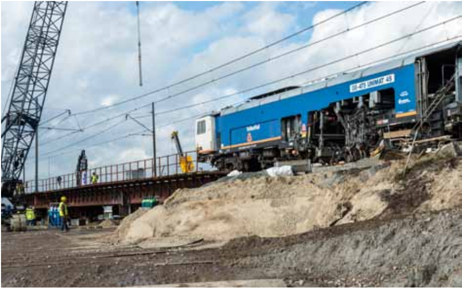
Figure 6.7: Temporary auxiliary bridge on the Amsterdam-Almere rail line (Photo: Rijkswaterstaat)
