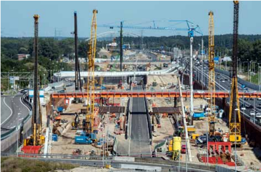
Figure 5.1: De Gaasperdammer Tunnel under construction (Photo: IXAS)
