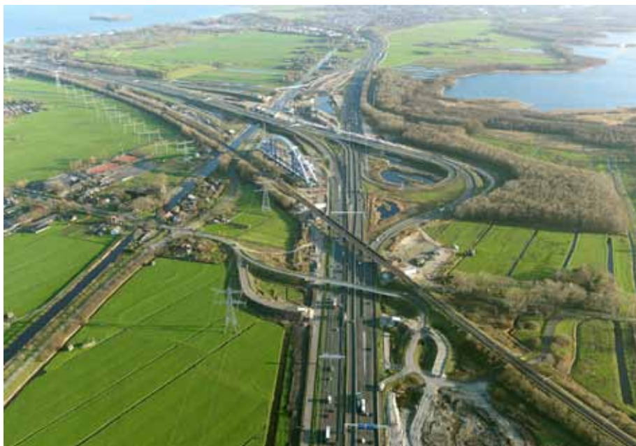
Figure 1.1: A construction site of the SAA infrastructure program (Photo: Rijkswaterstaat)
