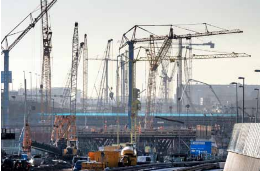
Figure 7.5: The construction of the Gaasperdammer Tunnel in full swing (Photo: IXAS)
